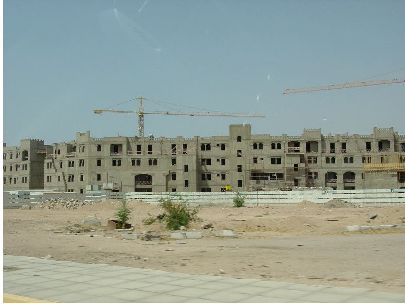
4.18 Construction site of Saraya Aqaba. Photo by author 2010.
